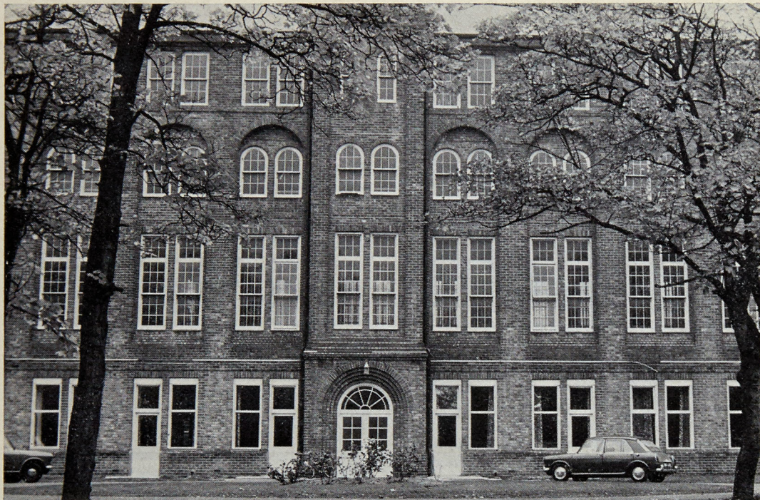
One side of the "FRESHFIELDS" complex. The ground floor, formerly class rooms, have been converted into bedrooms, lounges and day care rooms. The windows on the second floor are from the large assembly hall, which once a lift is installed will be available to the residents. Ack. The Southport Visitor
